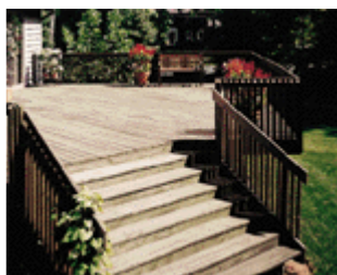
Before application of Spa-N-Deck
